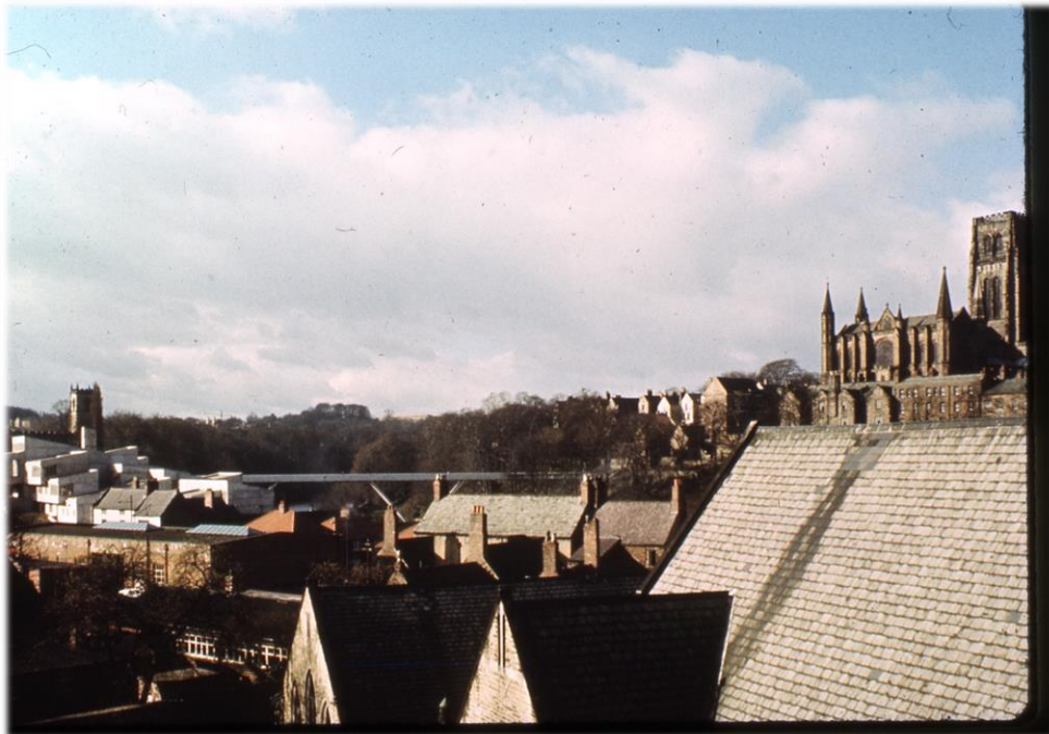
Dunelm House with Kingsgate Bridge linking to Durham Cathedral. The tumbling shapes of the town side elevations of Dunelm House were meant to match the vernacular architecture of Durham City.
